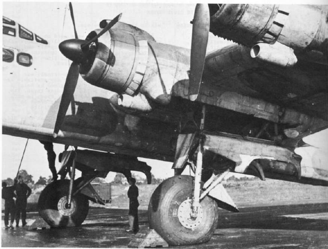
The massive and complicated undercarriage of a Stirling V
